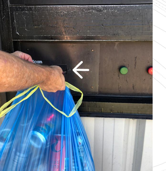
Place the scantron tag up to the scanner at the drop door site. The green light should go on and you will hear a click as the door is unlatched. Open the door and place your bag inside.
